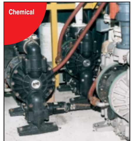
Non-metallic ARO pumps are used to move a variety of acids.
